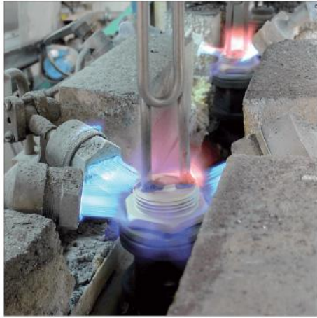
Brazing process at Backer OBR Sp. z o.o.
